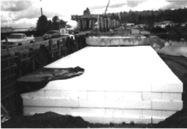
Figure 11.1 Geofoam. ( R-Control Building Systems )
