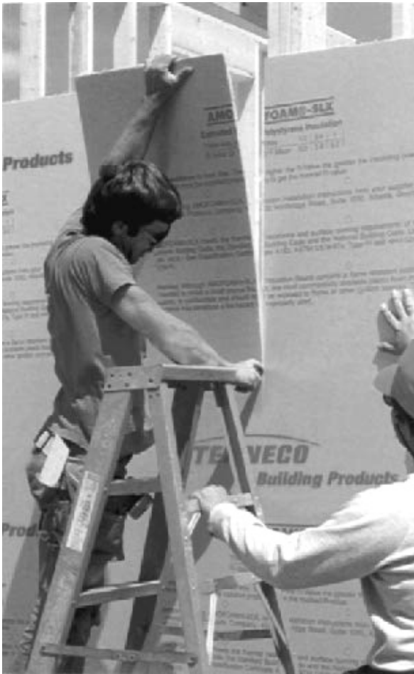
Figure 11.5 Extruded polystyrene. (Tenneco)
