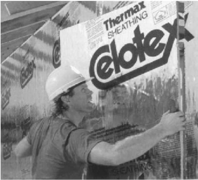
Figure 11.10 Foil-faced polyisocyanurate sheathing. ( Celotex )
