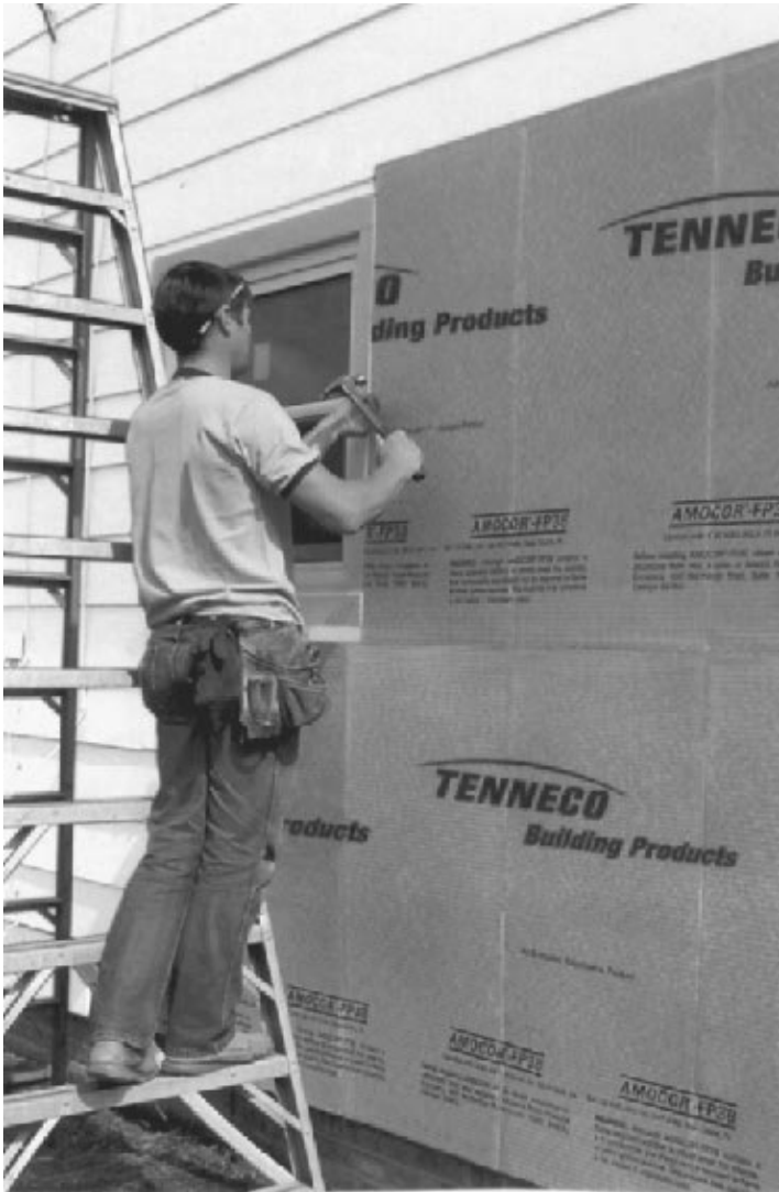
Figure 11.7 Residing underlayment. ( Pactive )
