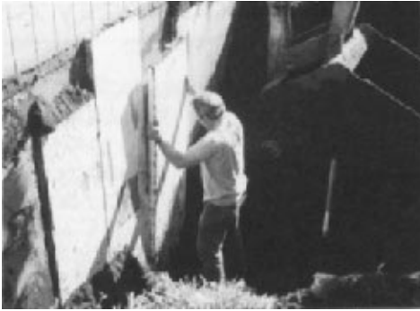
Figure 11.3 EPS below grade. ( R-Control Building Systems )
